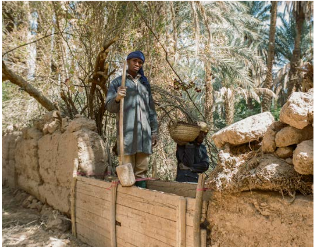
Ali is one of the last craftsmen in the Akka oasis to continue the traditional cob construction. February 2021.
